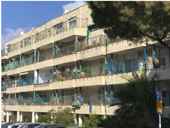
Fig. 3 Photograph of multi-unit apartment building in Jerusalem
